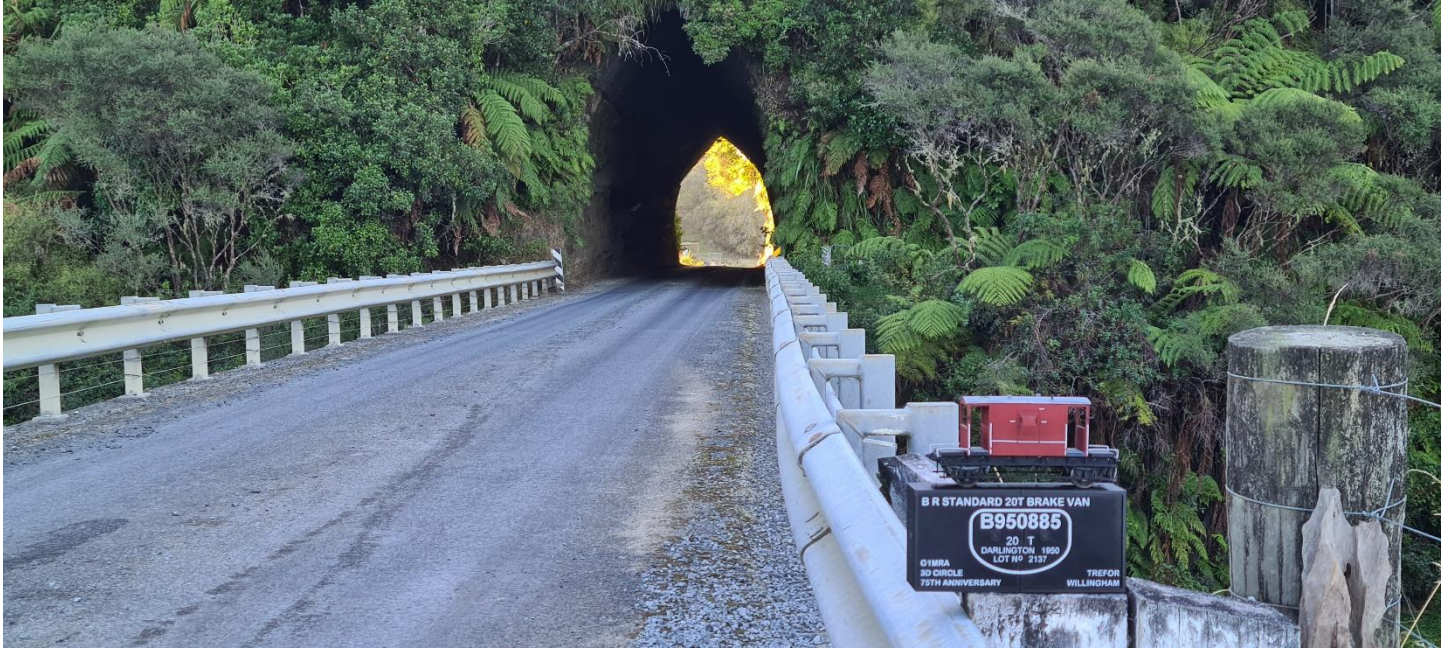
A closer view of the tunnel's unusual profile. The pointed invert is due to the shaly material it has been bored through which would not otherwise hold up if a normal arched profile was used. This follows a similar technique used for the railway tunnels through the chalk cliffs at Dover for precisely the same reasons.
