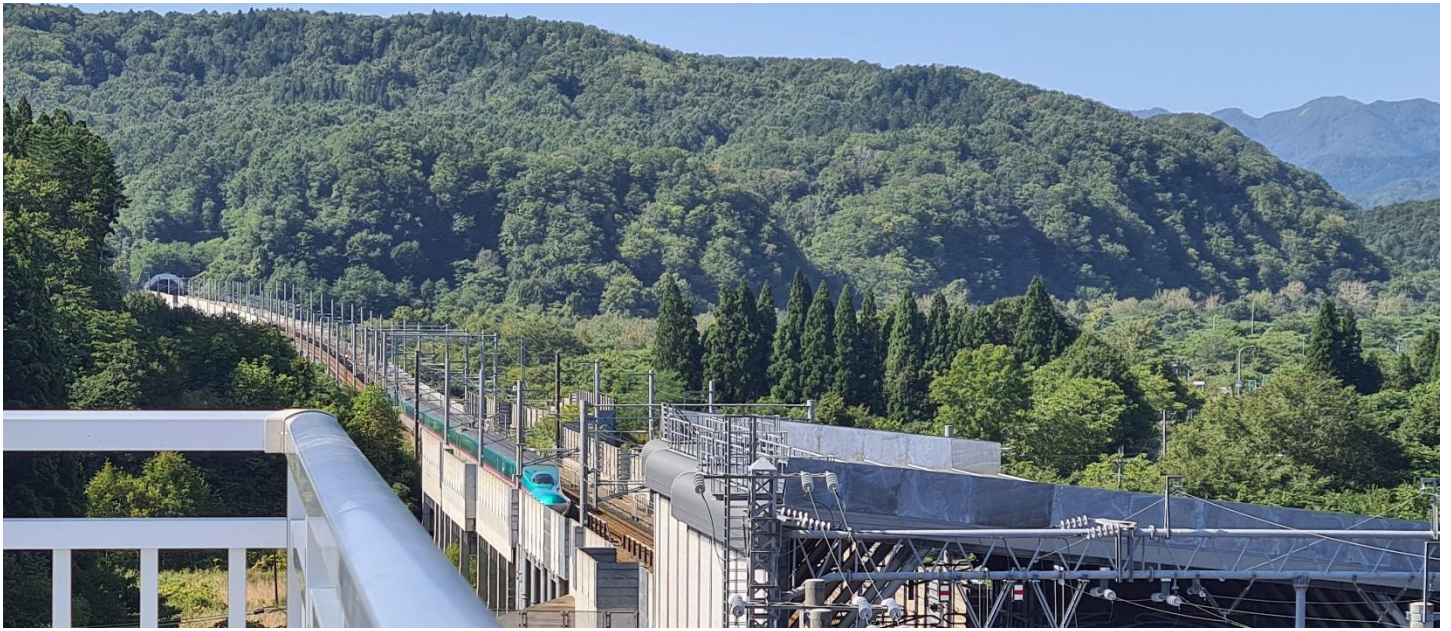
A Shinkansen heading for the tunnel and Honshu.
