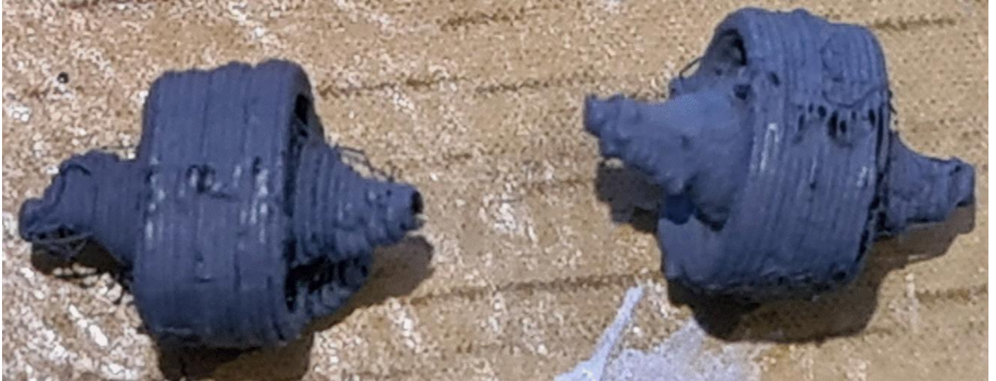
A rather cruel shot of the original roof ventilators.
